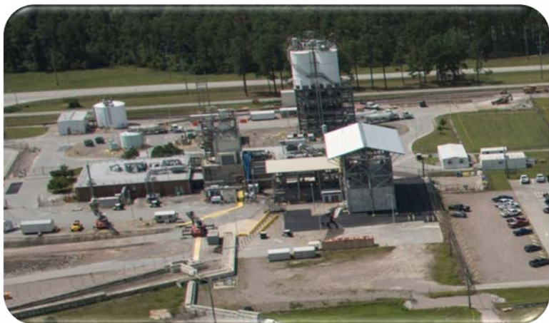
Saltstone Production Facility
