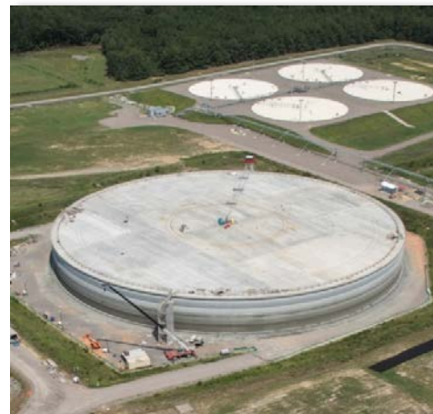
Saltstone Disposal Unit (SDU-6)
