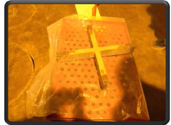
First Canister Support Crossbar Removed
