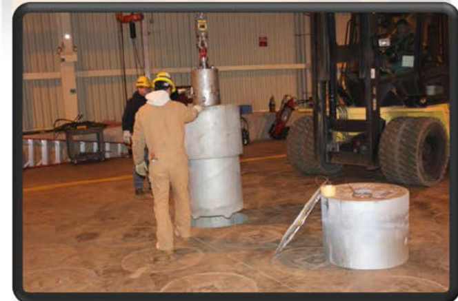
Shield Plug Replacement
