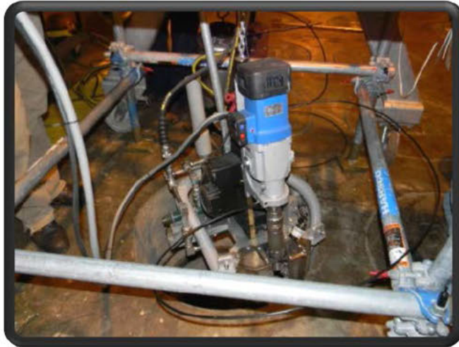
Crossbar Cutting Tool In Field
