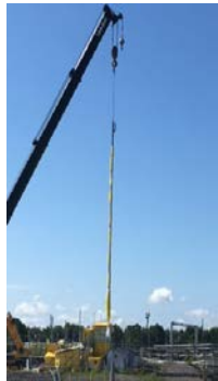
SRR TCCR Preparation Photos (Above)
