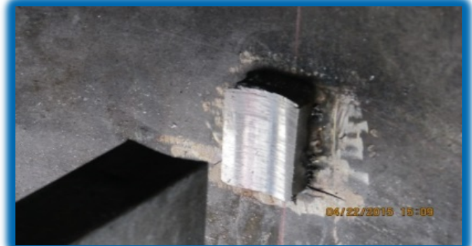
Completed Crossbar Cut
