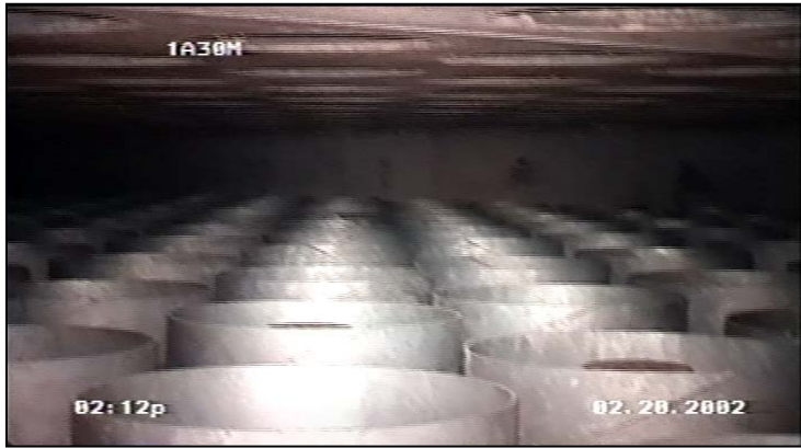
Inside View across vault A - Single Storage
