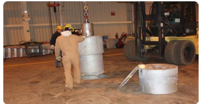
Concrete Plug being replaced with Redesigned Steel Plug
