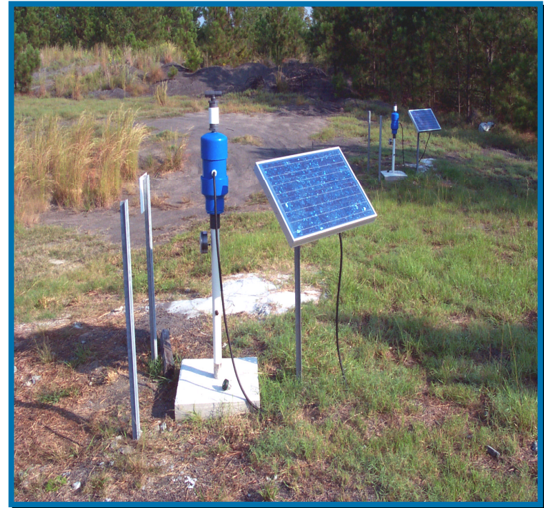
Typical Solar Powered MicroBlower Well
