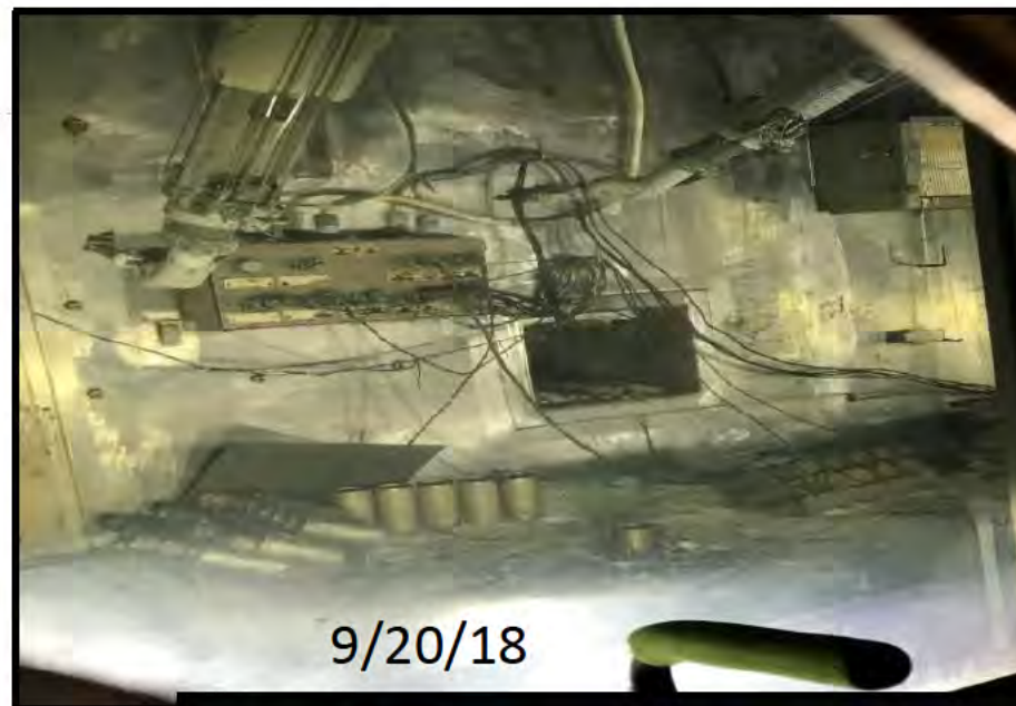
View of inside cell #1. Before & after MAR removal.
