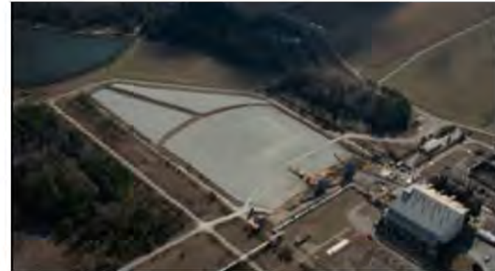
After: Aerial of End State of D Powerhouse Coal Pile Remediation
