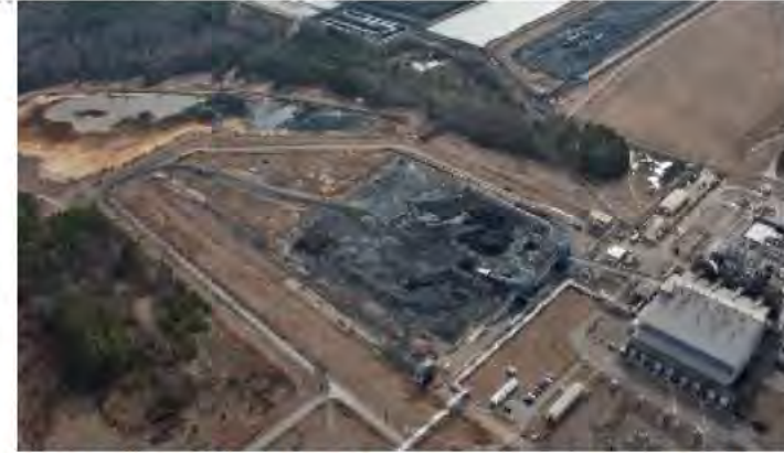
Before: Aerial of D Powerhouse Coal Pile Remediation
