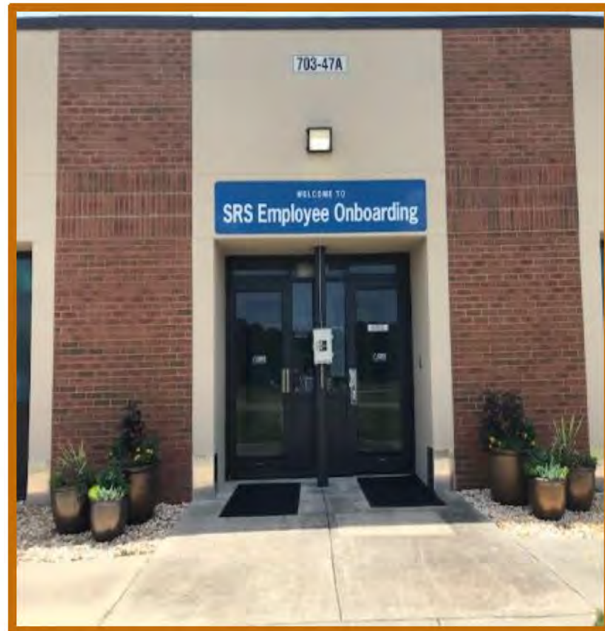
703-47A Renovated Exterior (After)
