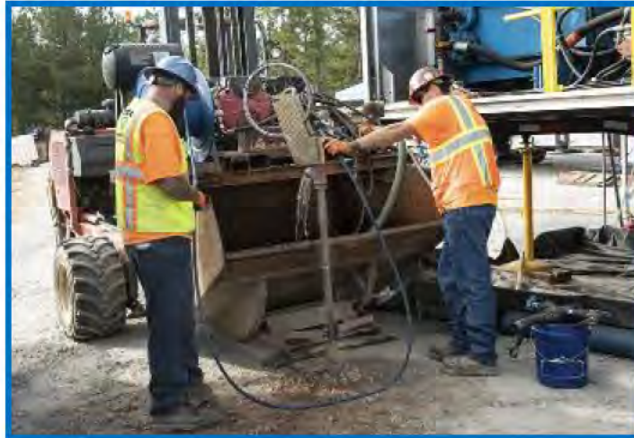
Permeable Reactive Barrier Injection
