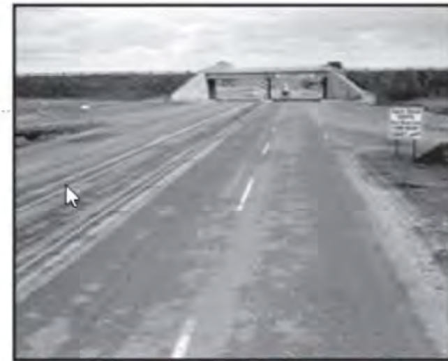
View of Cloverleaf Intersection, February 11, 1952, SRS Negative M621
