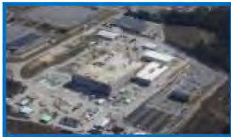
Pu Processing Facility (NNSA)
