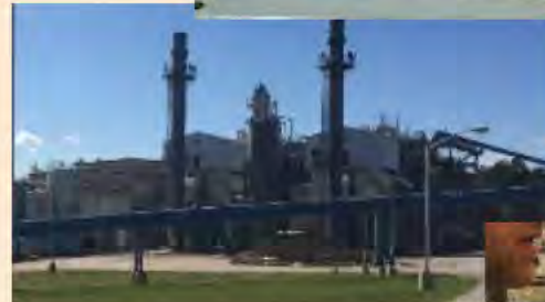
Biomass Plant (Steam)
