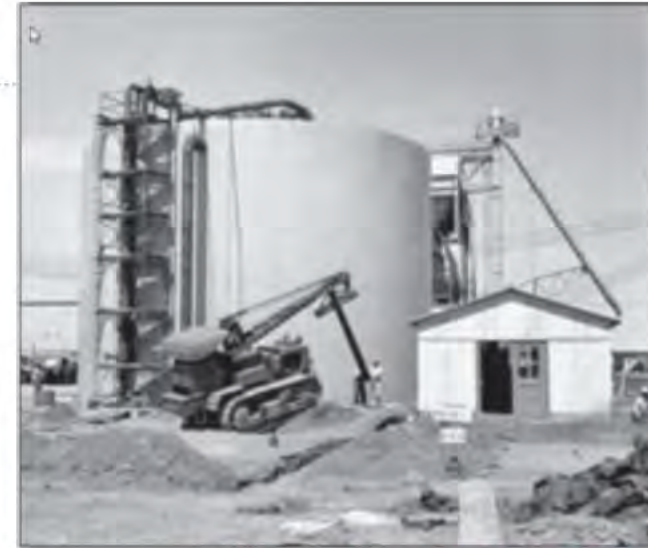
782-A Reservoir Construction, August 28, 1952.
