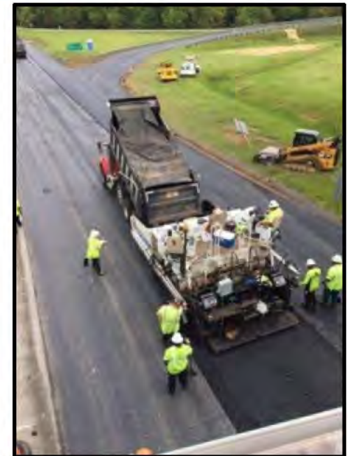
Road C Repaving
