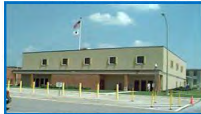
703-46A SRS Badge Office Refurbishment Complete 2019
