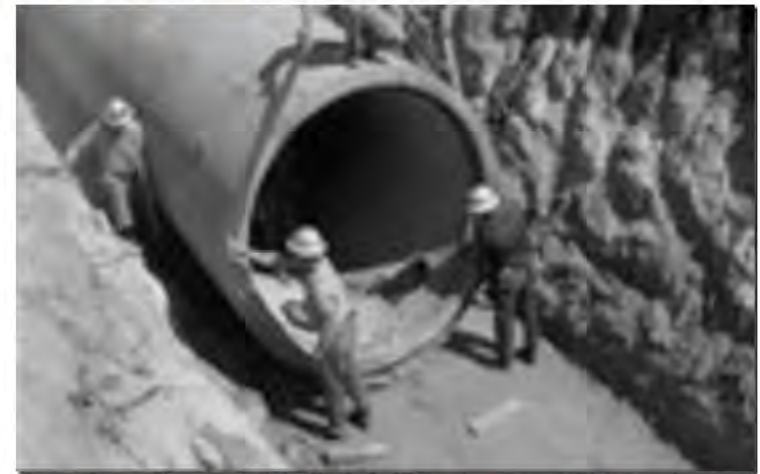
Laying Water Lines, April 3, 1952, SRS Negative DPESF-712-08
